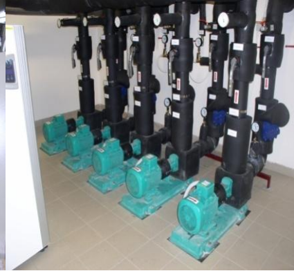
Fig. 2. Circulation Pumps in Primary Circuit
