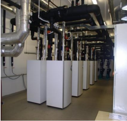
Fig. 1. Heat Pumps - 10 units
