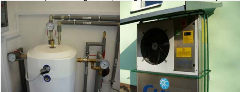
Fig. 2. Current unsatisfactory status of heating installation.
