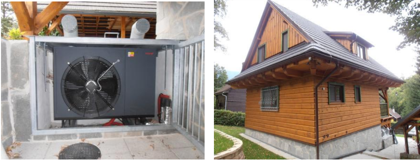
Fig 1. Installed heat pump and heated object. (Šrámek,2012)
