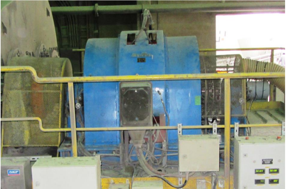
Fig. 1. Motor of a mill in a cement plant, that is three-phase induction slip-ring motor DOLMEL SYUe-148r/01 type, with power of P_N = 1000 kW, n = 738 rpm.
