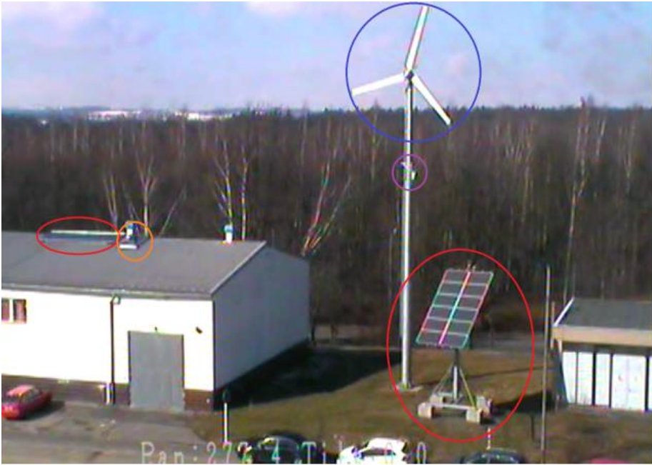
Fig. 2: Print screen from Security System with Marked Components of Hybrid System
