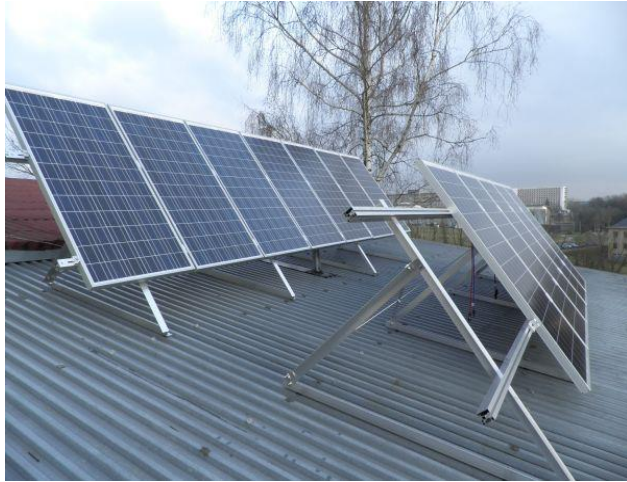
Fig. 1. Small photovoltaic power plant on the roof of laboratory
