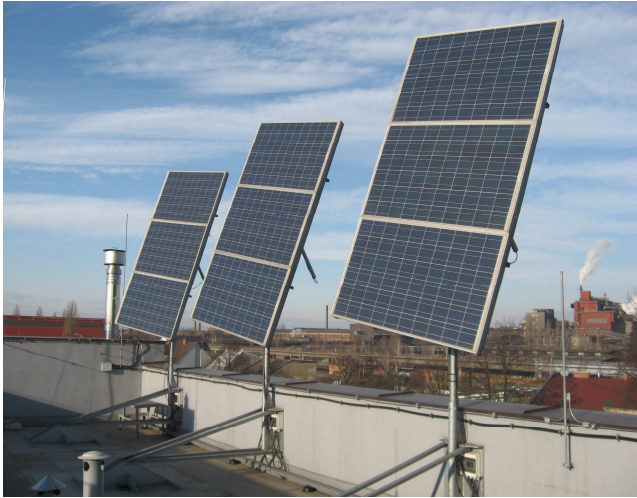
Fig. 1. Photovoltaic panels of the second section
