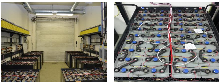
Figure 4 Battery room and main storage battery
