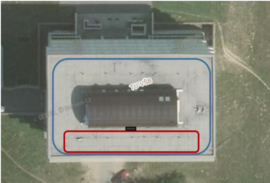
Fig. 1. Placement of the cable polygon on the roof of the N building.
