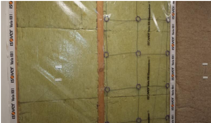
Fig. 2. Placement of the third sensory layer and waterproof membrane
