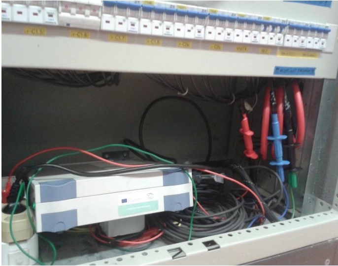
Fig. 1. Connected measuring device in distributor.
