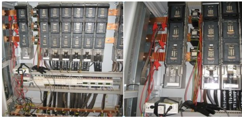
Fig. 1. Demonstration of connection measurement equipment in the BS 1
