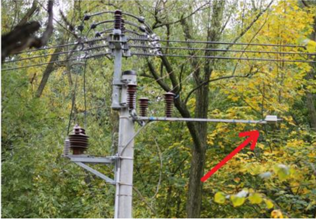
Fig. 4. BONI whip antenna mounted on the pole
