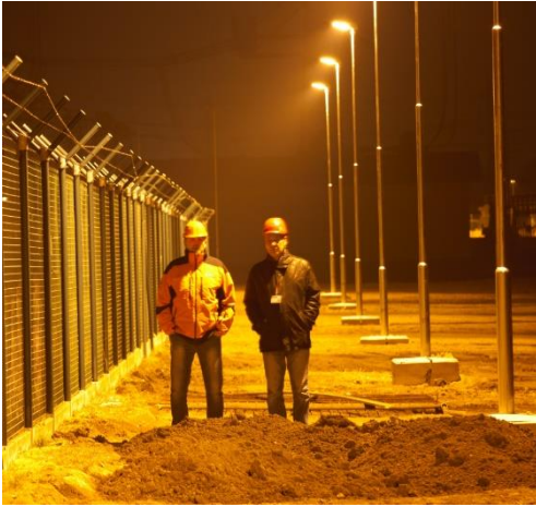
Fig. 2. Watchdog lighting system in the area of electric station
