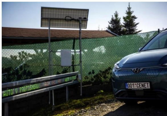
Fig. 7. Current version smart crash barrier located in Suche Lazce
