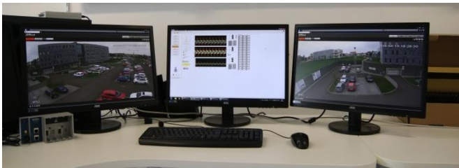
Fig. 2. The control room
