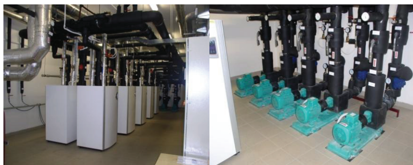
Fig. 1. Heat pumps, 10 units Fig. 2. Circulating pumps within the primary circuit
